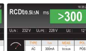
Test on RCDs.
