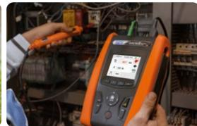
Start/stop measuring with remote lead PR400.
